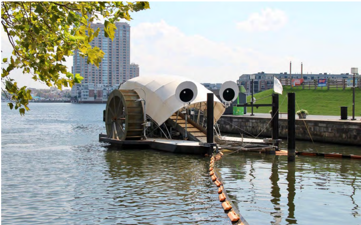
Figure 8-5: In Baltimore, a trash interceptor device named "Mr. Trash Wheel" captures people's hearts as it captures trash floating down the Jones Falls River before entering the Inner Harbor
