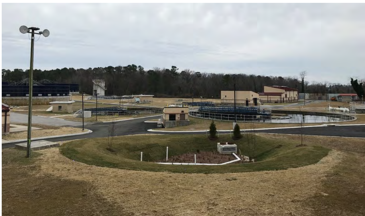
Figure 8-2: Salisbury's Wastewater Treatment Plant
