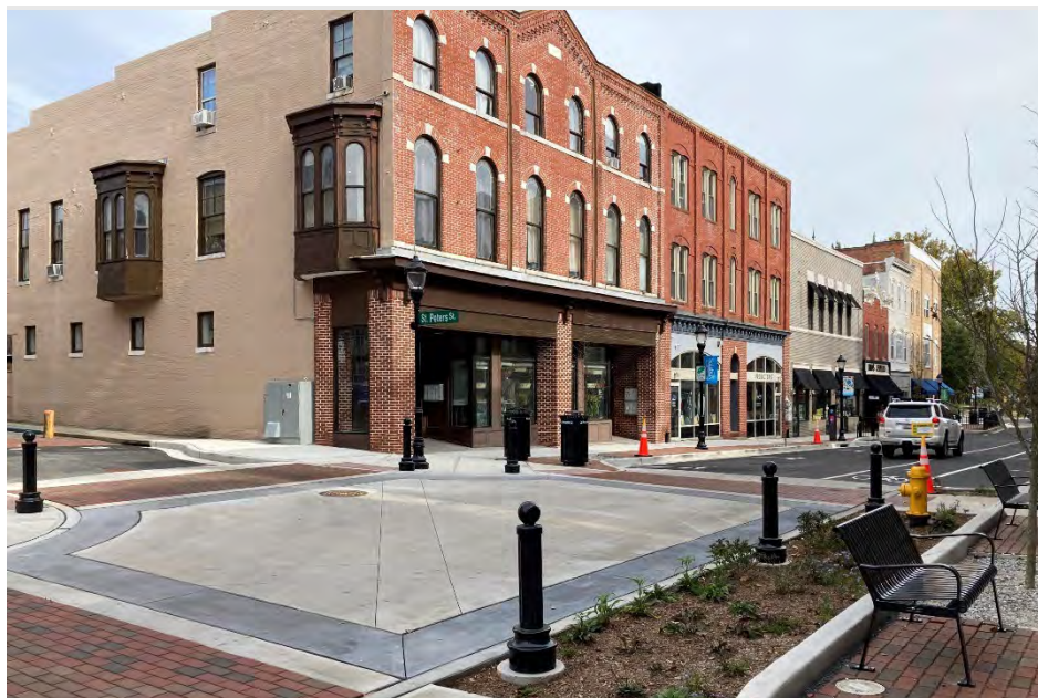
Figure 6-1: Recently reconstructed streetscape on Main Street in downtown Salisbury has created a more attractive and welcoming area for local business patrons with traffic calming to reduce speeding and improve safety.
