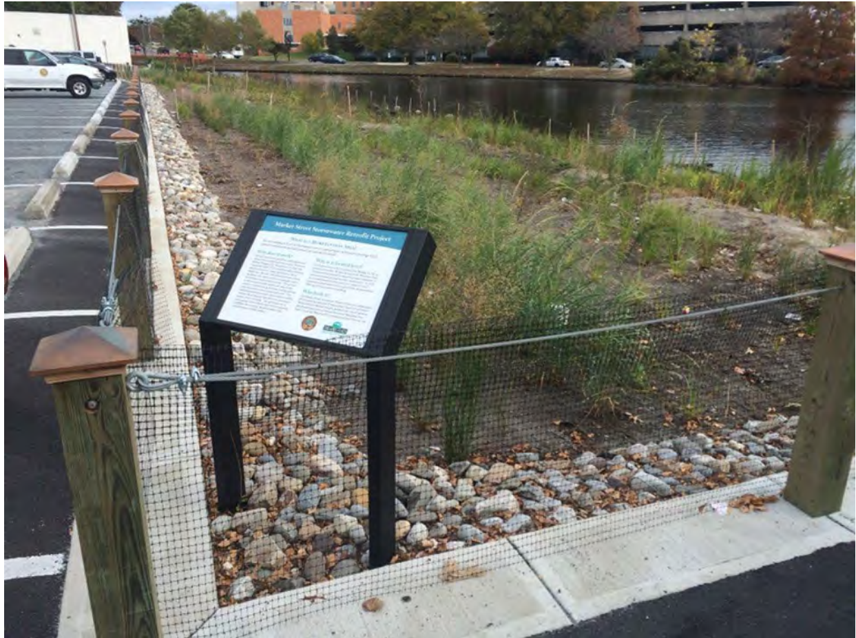
Figure 8-4: Shoreline improvements along the Wicomico River with bioengineered green infrastructure helping to improve water quality, stabilize the shoreline soils, and create a natural habitat for local pollinators and wildlife.
