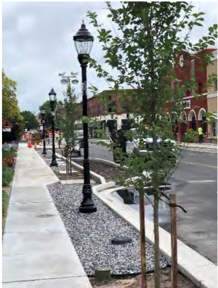
Figure 9-2: During construction of Salisbury's Main Street, the design included extensive tree wells and bioretention systems to increase tree canopy and infiltrate stormwater runoff. These are important strategies to a more sustainable and resilient future.
